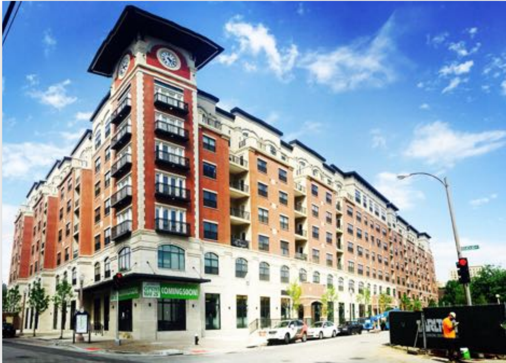
The Orion Whole Foods, 177 Apartment Units, and 438 space parking garage
